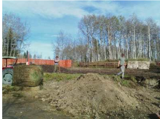
Removing existing corral fencing.
